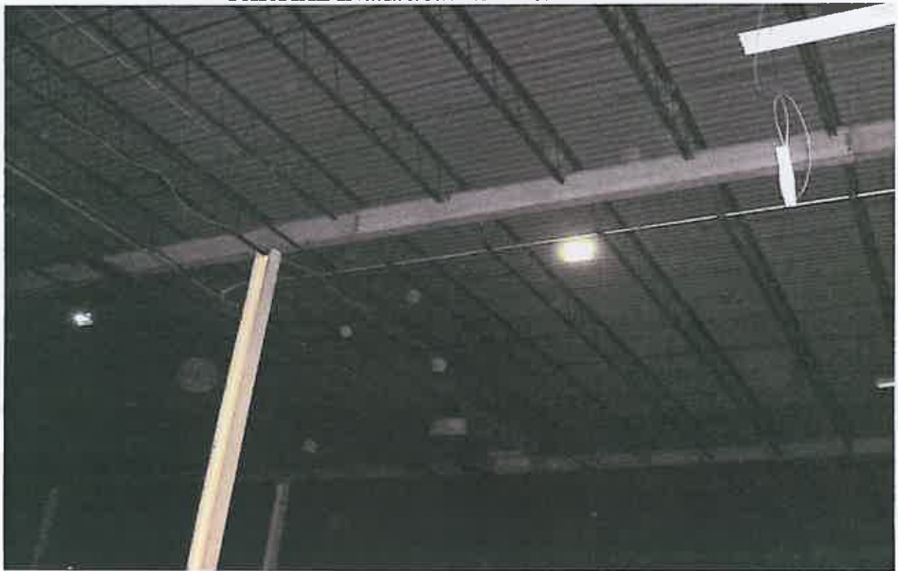
PARTIAL INTERIOR VIEW OF CEILING OF SUBJECT
