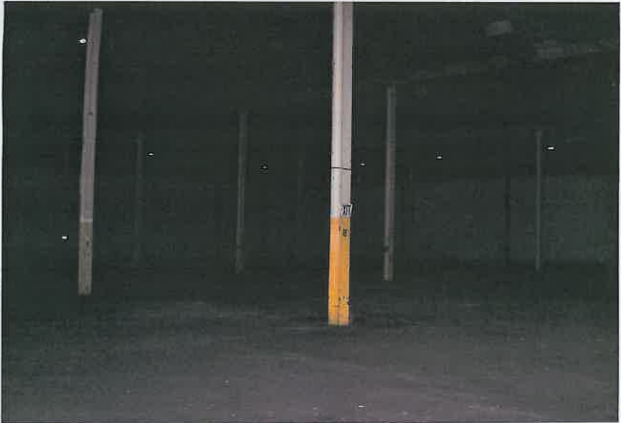
PARTIAL INTERIOR VIEW OF SUBJECT
