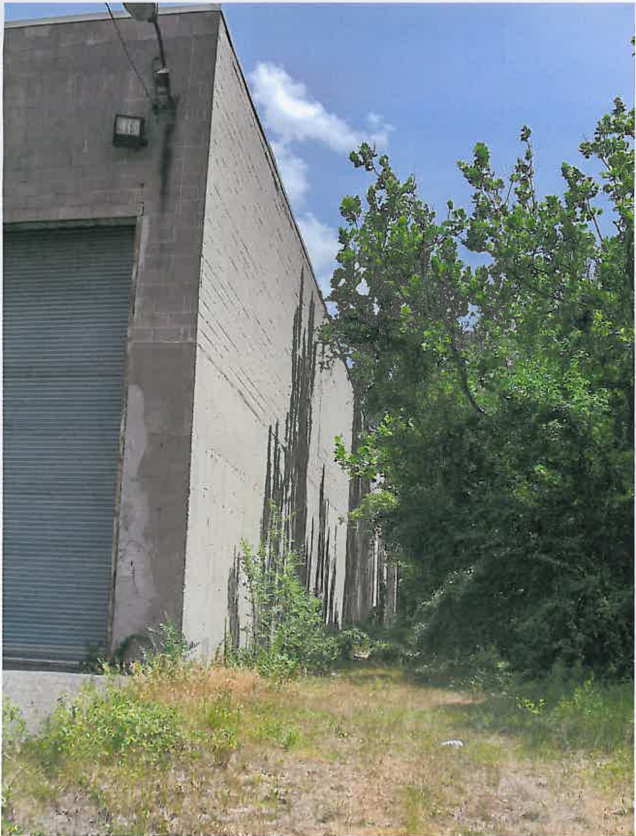
REAR ELEVATION OF SUBJECT, CAMERA FACING SOUTHERLY
