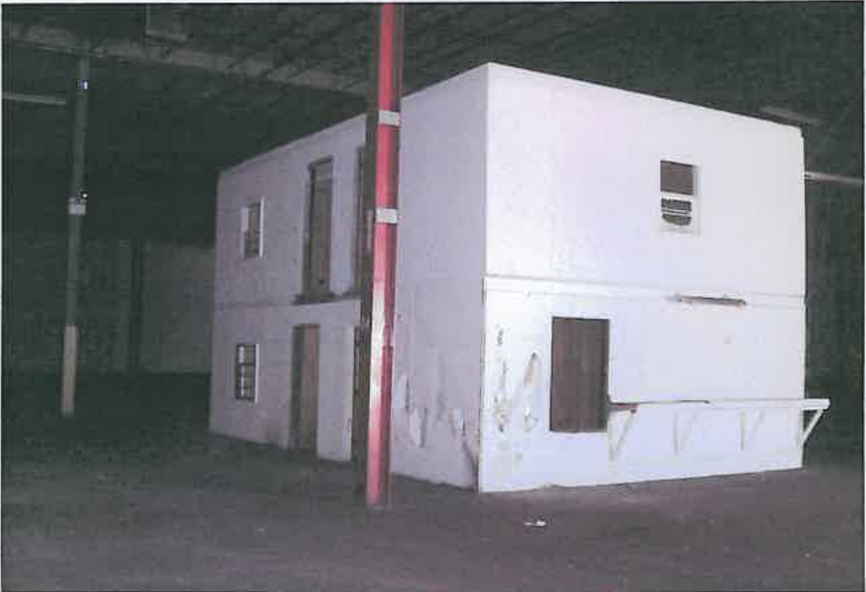
PARTIAL INTERIOR VIEW OF FORMER OFFICE AREA OF SUBJECT
